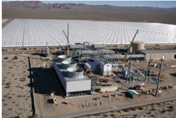
Acciona Solar's $110 million, 54 MW solar power plant in Nevada ACCIONA
